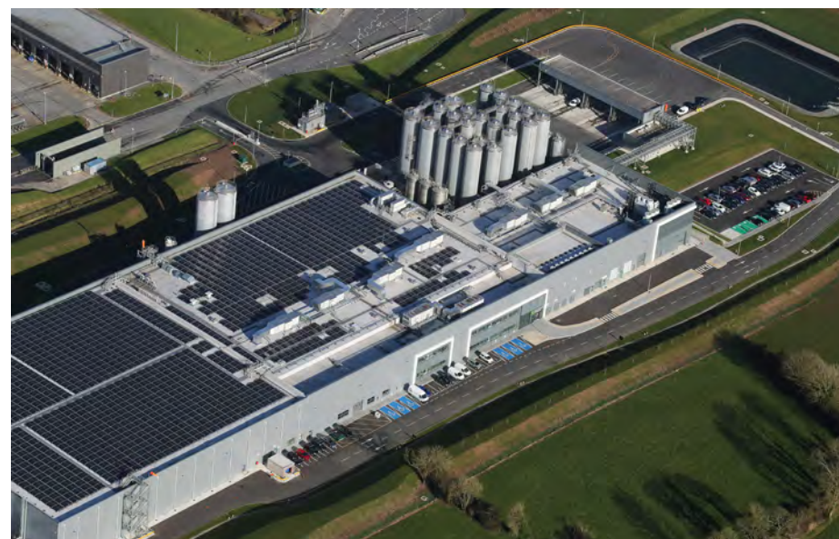
Aerial view of Kilkenny Cheese manufacturing facility at Belview, South Kilkenny.
